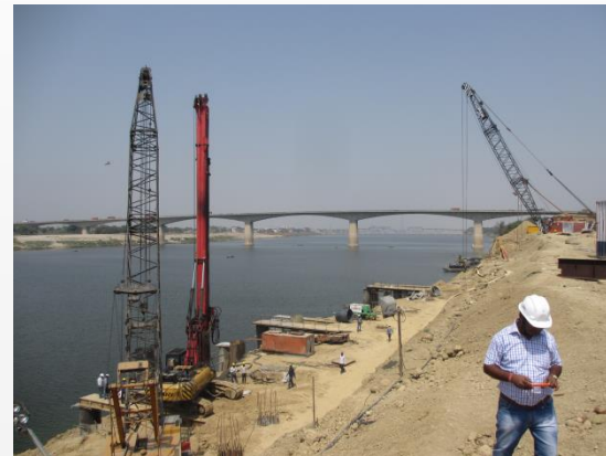
Varanasi - construction of the jetty Photo Wagener
