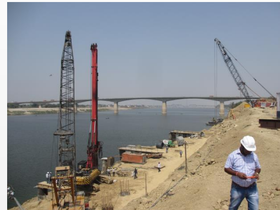
Varanasi - construction of the jetty Photo Wagener
